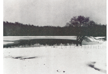
TROY, NC – Ten-acre Oxidation Pond for treatment of sewage.
