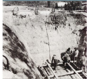
GEORGETOWN, SC – Excavation for sewage pumping station. Also begun in the 1950s, this site was one of five planned for the sewer system of the "Maryville Section" which was eventually annexed to the City of Georgetown in 1957.
