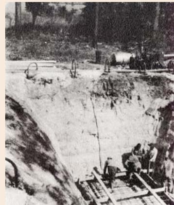
*GEORGETOWN, SC – Excavation for sewage pumping station. Also begun in the 1950s, this site was one of five planned for the sewer system of the "Maryville Section" which was eventually annexed to the City of Georgetown in 1957. W.K. Dickson's project description made special mention of "...the use of the Well Point System to control ground water during construction."*
