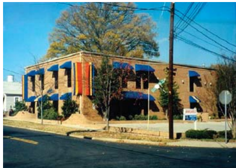
Former office space at 1924 Cleveland Avenue.
