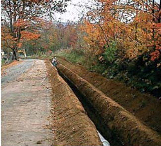
Sewer-line installation for Charlotte Mecklenburg Utilities.
