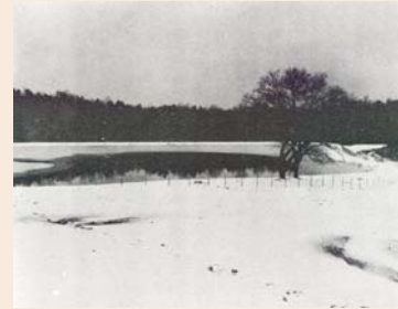
TROY, NC – Ten-acre Oxidation Pond for treatment of domestic sewage. This plant began operation in the late 1950s. According to W.K. Dickson marketing material of the time, "...the lagoon has been free of odors and has provided treatment for the waste of a quality meeting the requirements of Health Authorities and provides an attractive habitation for ducks."
